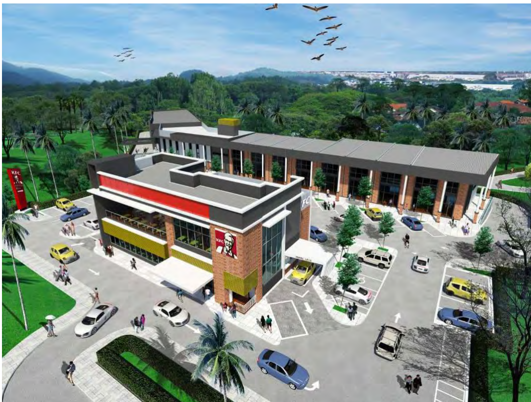
8 Units Shop, Multi-Purpose Hall & KFC Restaurant (Mixed Development) Client: Laman Baiduri Sdn Bhd Site : Bandar Taiping Status: On Going
