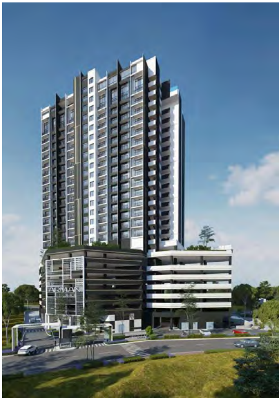
319 Units 26-Storey Soho Building Client: Erayear Properties Sdn Bhd Site : Tmn Perindustrian Sime UEP Status: On Going
