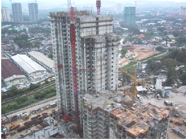
1022 Units 37-Storey Apartment Client: Mayland Development Sdn. Bhd Site : Jalan Kuching Status: Completed (Contractor's Alternative Design)
