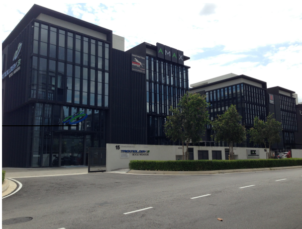
10 Units Semi-D Factory At Kota Damansara
