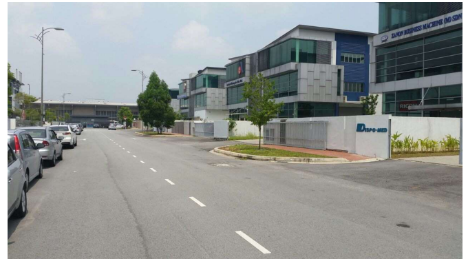
18 Units Semi-D Factory At Kota Damansara
