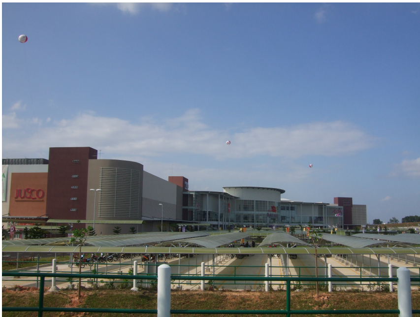
3-Storey Shopping Complex (Jaya Jusco Shopping)
